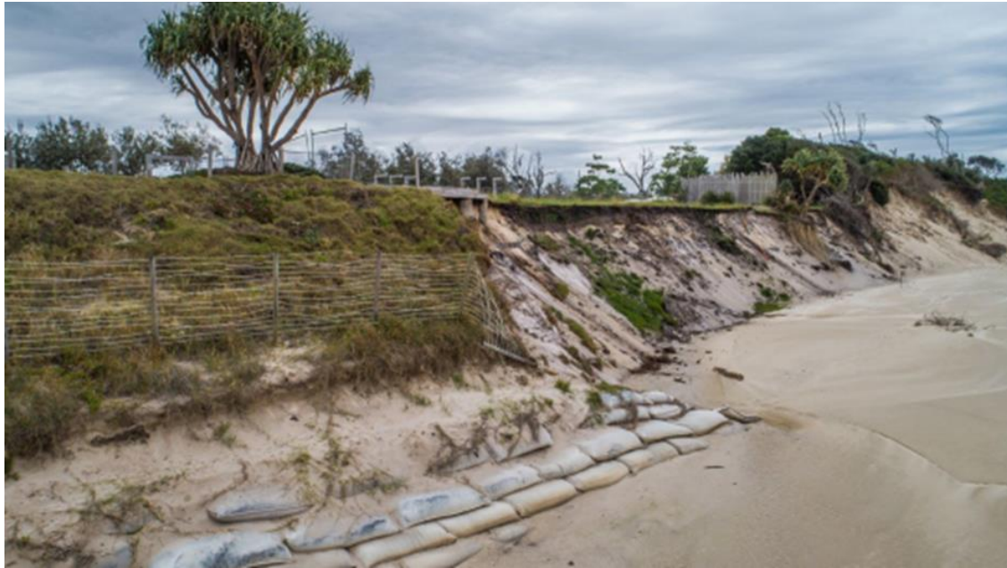
Figure 1: Existing geobag wall in foreground; site of proposed extension to the right (source: Coastal Engineering Assessment, Royal HaskoningDHV, May 2023)
