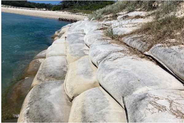
Figure 7: Existing geobag wall
