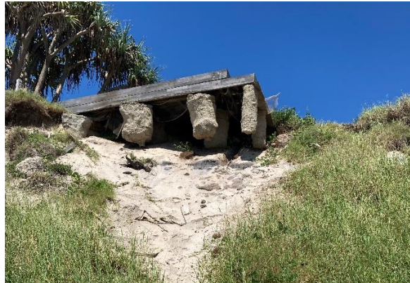
Figure 8: Viewing platform undermined by existing erosion
