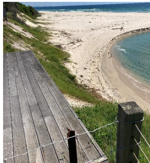
Figure 4: Erosion at western end of existing geobag wall
